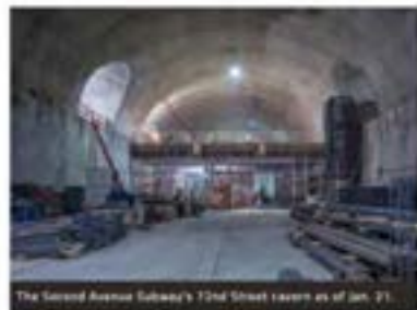
The Second Avenue Subway's 72nd Street cavern as of Jan. 21.
