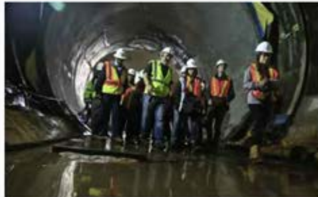
Second Avenue subway's 72nd St. station work falling behind
